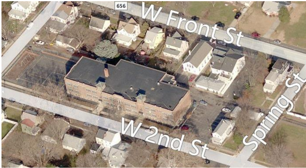
Figure 2- Aerial View of Duffy School
